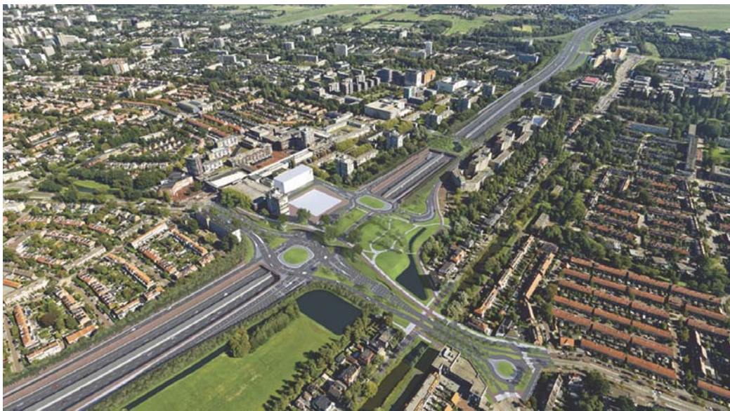
Photo 1 - Overview of A9 motorway near Amstelveen after reconstruction.
