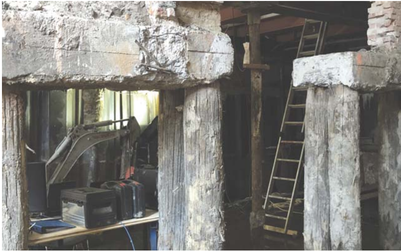
Figure 2 - Inspection of an Existing Timber Pile Foundation.
