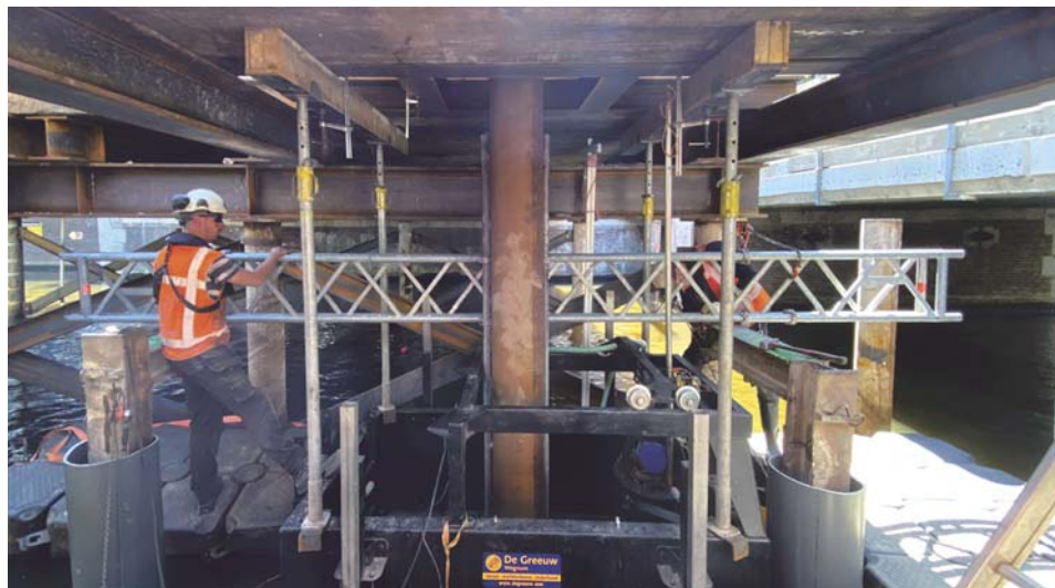
Photo 1 – Test installation below bridge deck.
