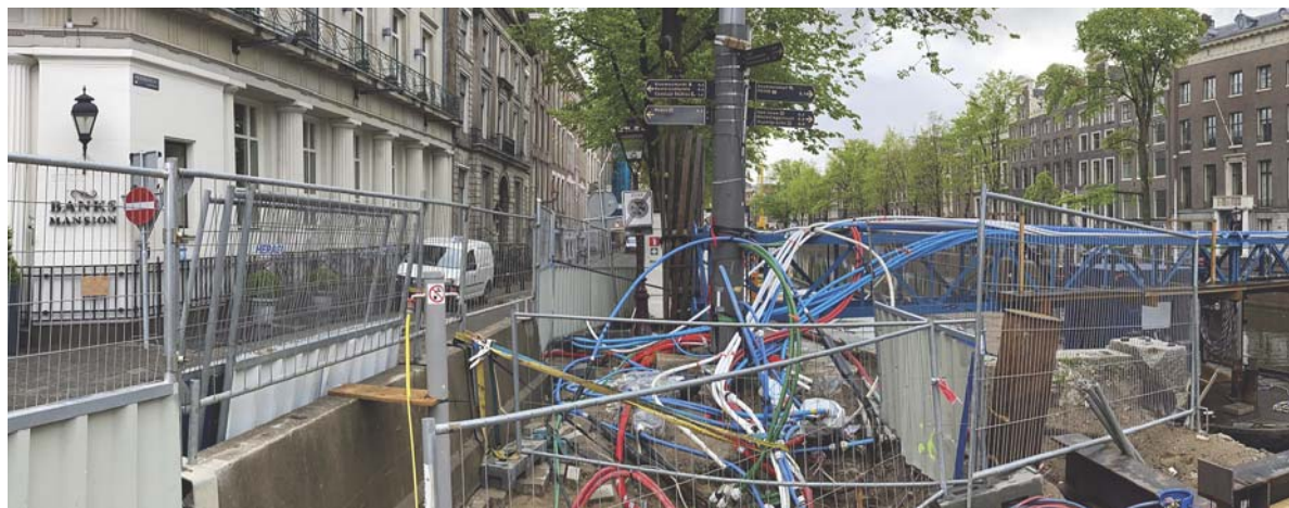
Photo 2 – Bridge deck abutment at street level.
